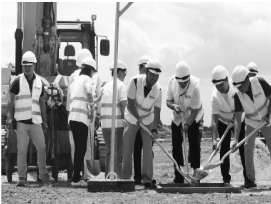
CALAEX GROUNDBREAKING. Public Works and Highways Secretary Mark Villar (left) and Cavite Governor Jesus Crispin Remulla (3rd left), lead the groundbreaking of the CALAEX Cavite Segment at the MPT South Headquarters Ground, Barangay Alapan II-B in Imus, Cavite on Wednesday (March 27, 2019). The Cavite Segment starts from Kawit and will traverse the Imus Open Canal, Governor’s Drive, Dasmariñas, Aguinaldo Highway, and Silang town. This will connect to the Laguna Segment of Sta. Rosa exiting to Mamlasan, Binan, Laguna towards SLEX. (PNA photo by Avito C. Dalan)
