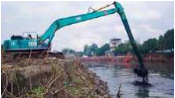
SMC's river cleanup initiative has returned to Tullahan River to restore its depth and carrying capacity for floodwater.
